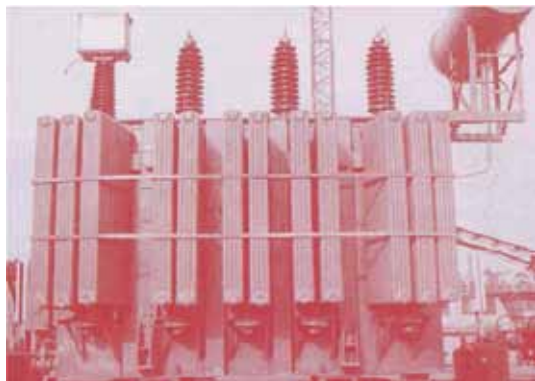
Rys. 4. Transformator 16 MV·A, 110 kV, 1953 r.
